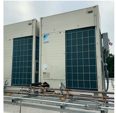
Clean HVAC coils on both outdoor and indoor equipment.
